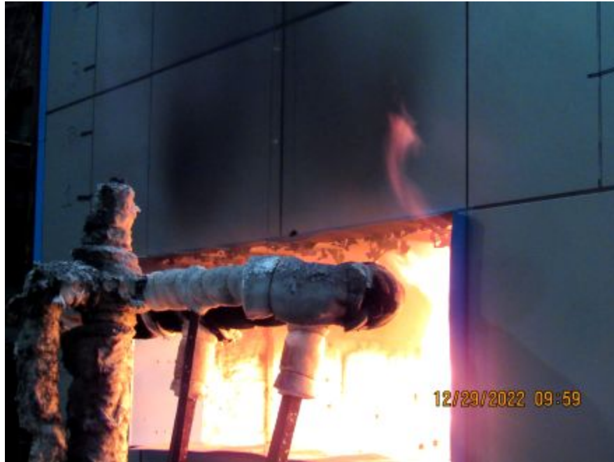
Photo No. 15 Flames exiting window opening
