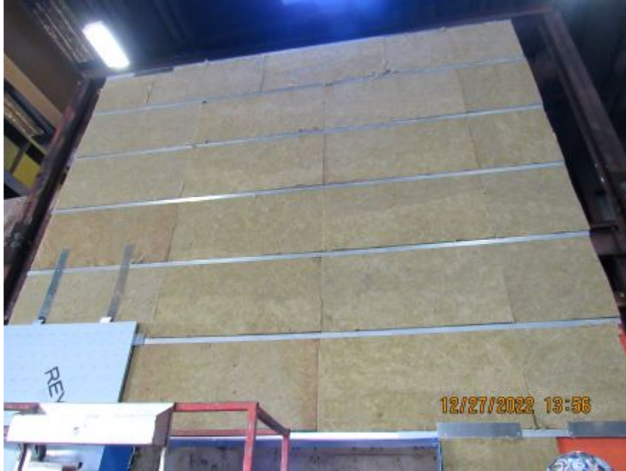
Photo No. 9 Mineral wool installed
