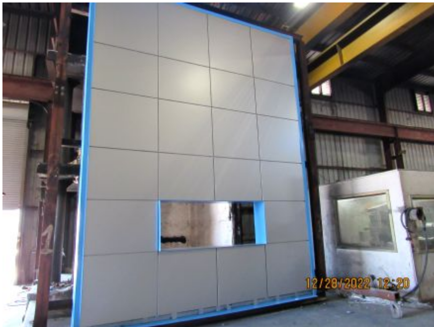
Photo No. 12 Wall assembly completed
