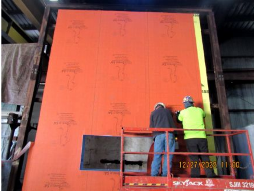
Photo No. 7 Installing vapor barrier
