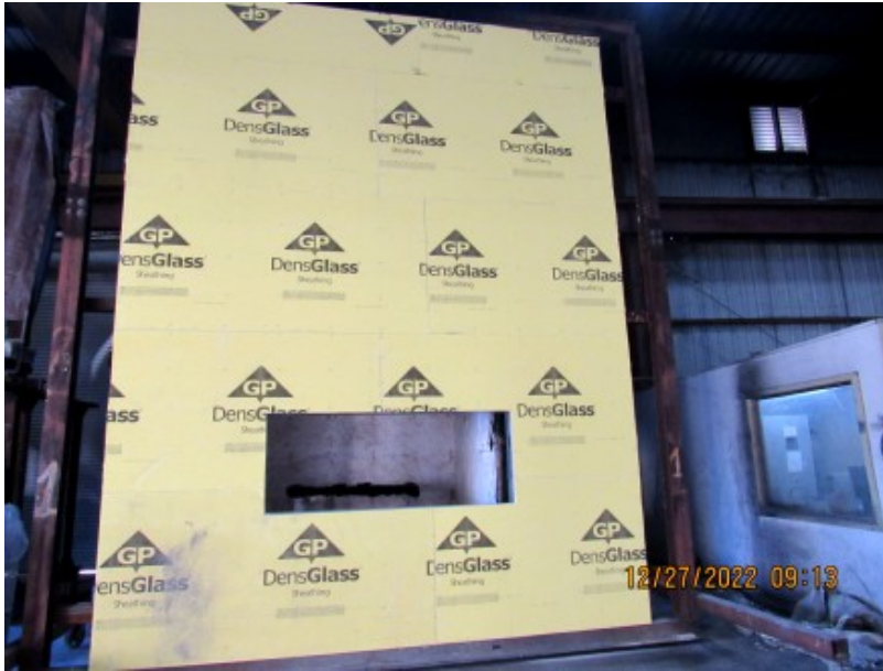
Photo No. 1 Base Wall
