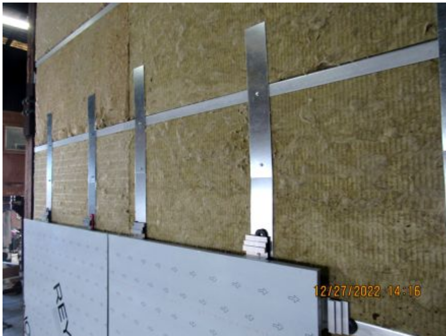
Photo No. 10 Installing panels with support steel strapping
