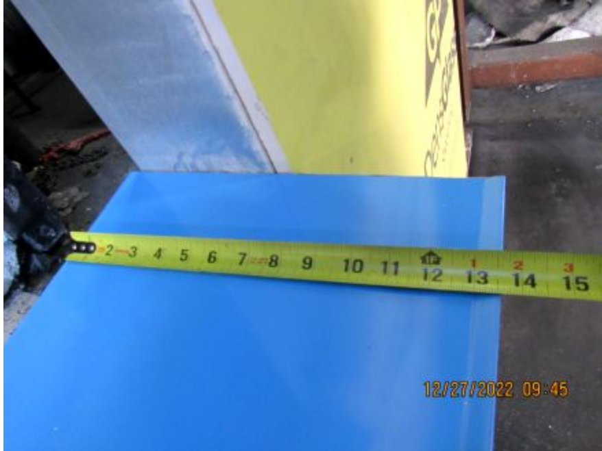
Photo No. 5 Window flashing
