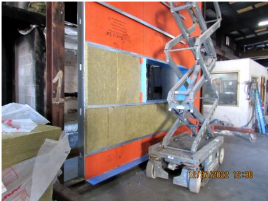
Photo No. 8 Installing zee girts and mineral wool
