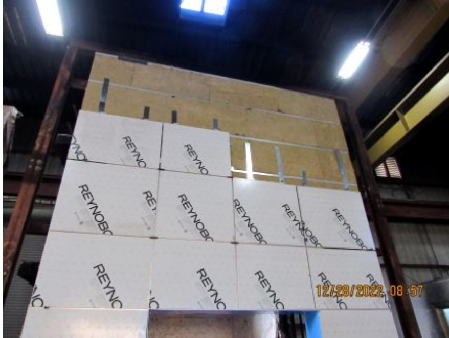
Photo No. 11 Panel installation continued
