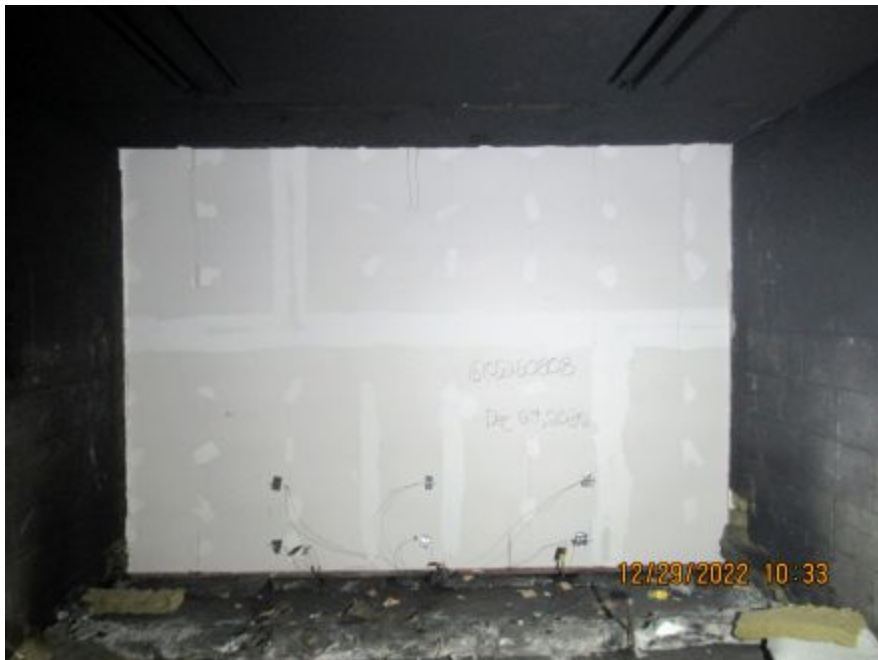
Photo No. 22 2 nd story back of wall post-test
