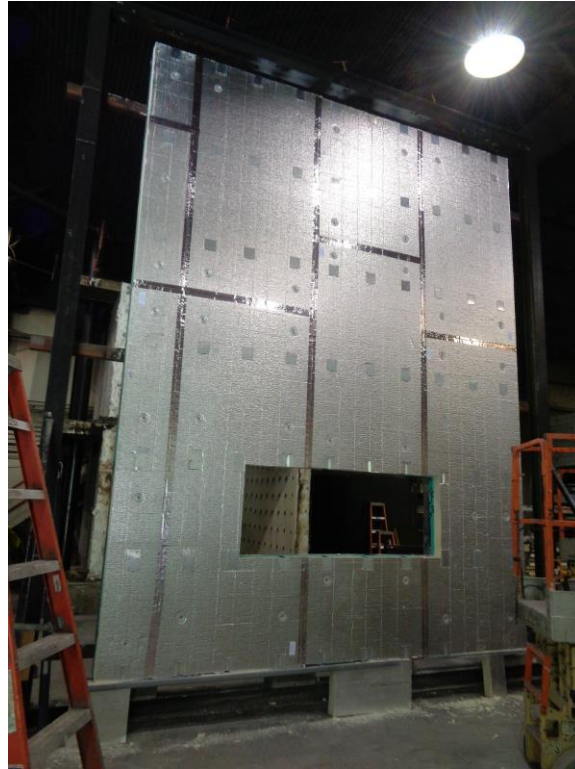
Photo No. 3 Installed Insulation and Technoform TE Hybrid Thermal Spacers
