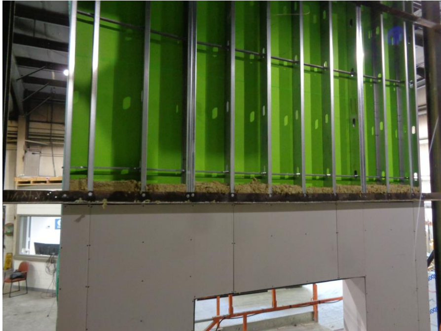
Photo No. 1 Core Wall Construction
