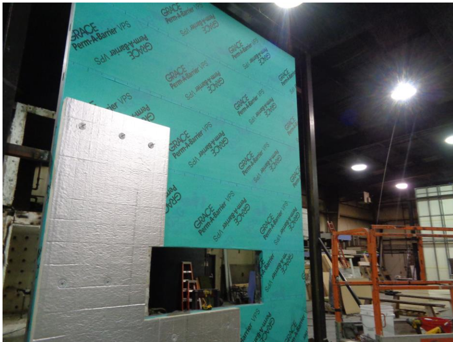
Photo No. 2 Installation of Grace Perm-A-Barrier® VP
