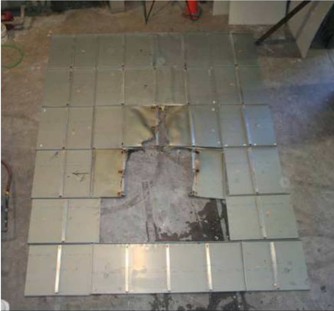
Figure B-15. Post-Test Assembly Dissection. Interior Surface of Reynobond Zinc Composite Material (ZCM) Panels.
