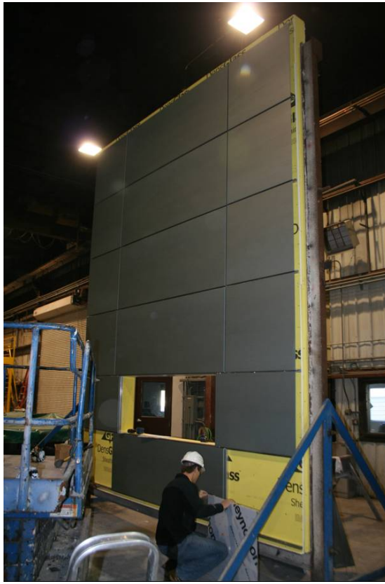
Figure B-1. Installation of the Reynobond Zinc Composite Material (ZCM) Panels.
