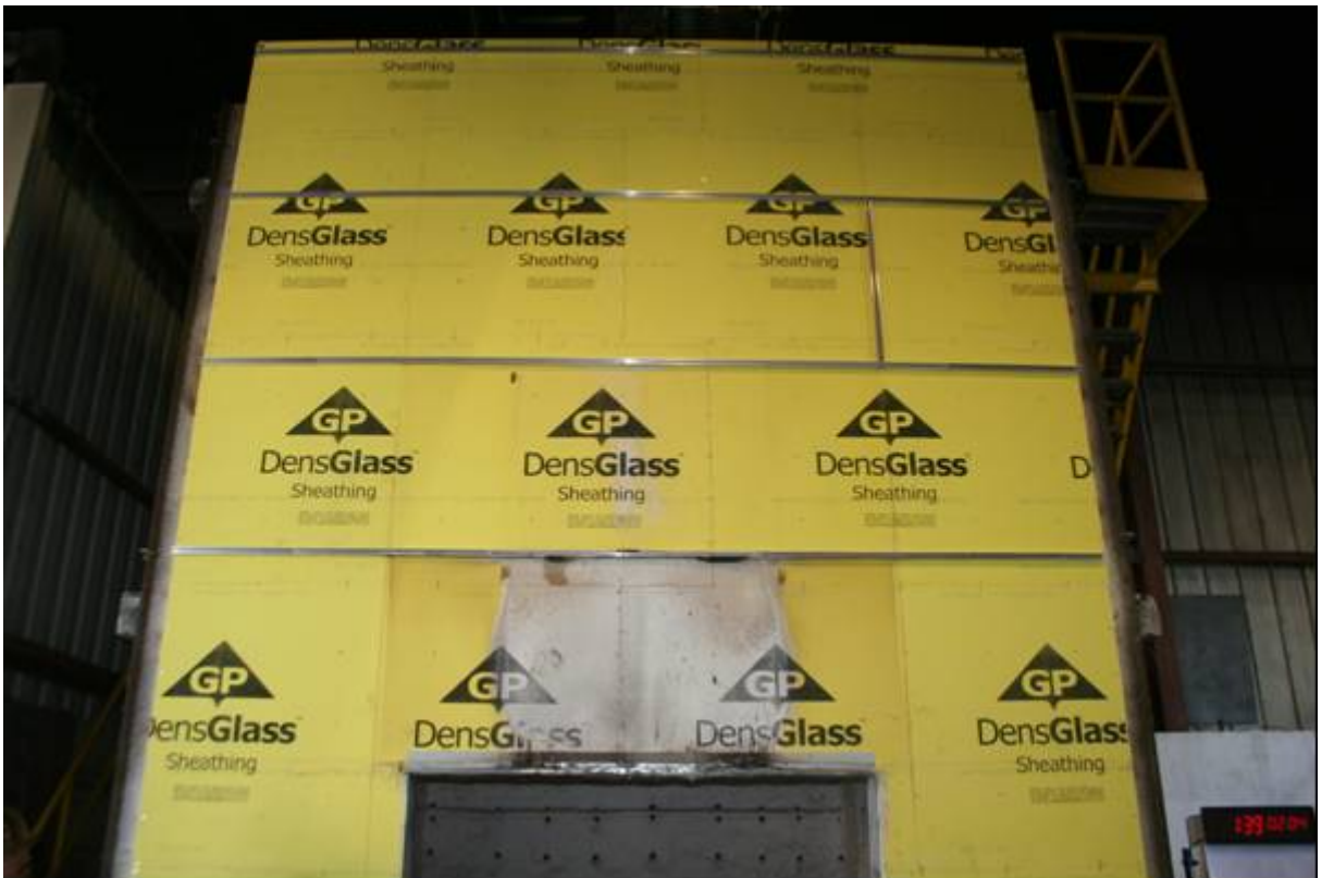
Figure B-14. Post-Test Assembly Dissection. Condition of Exterior Surface of Base Wall Underneath Panel System.
