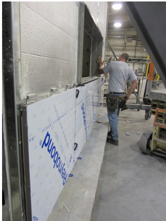
Photo No. 8 Panel Installation www.archtest.com
