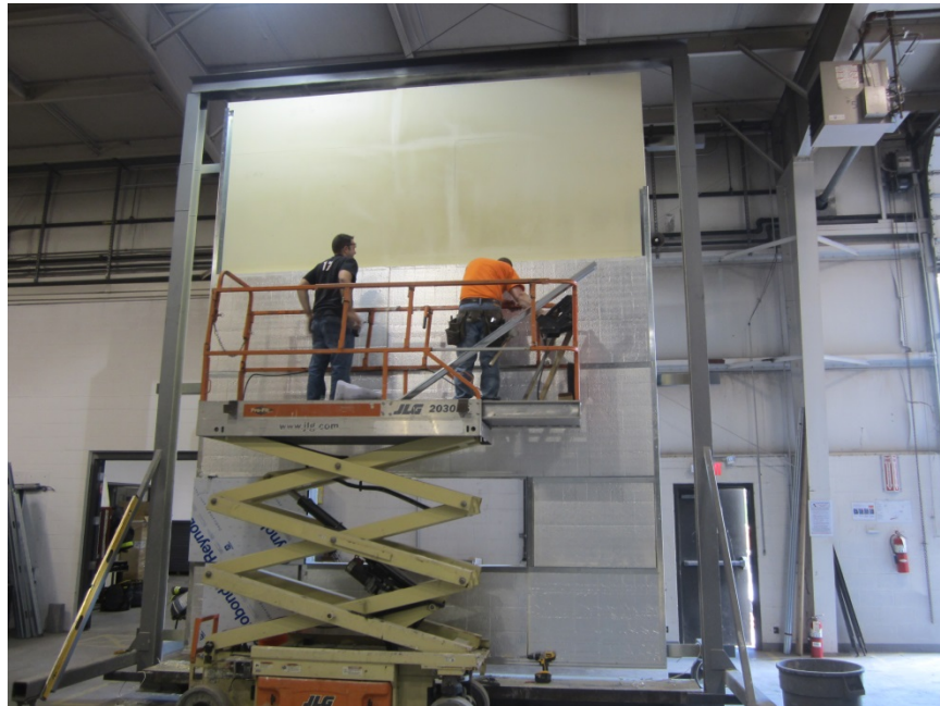
Photo No. 6 Insulation Installation
