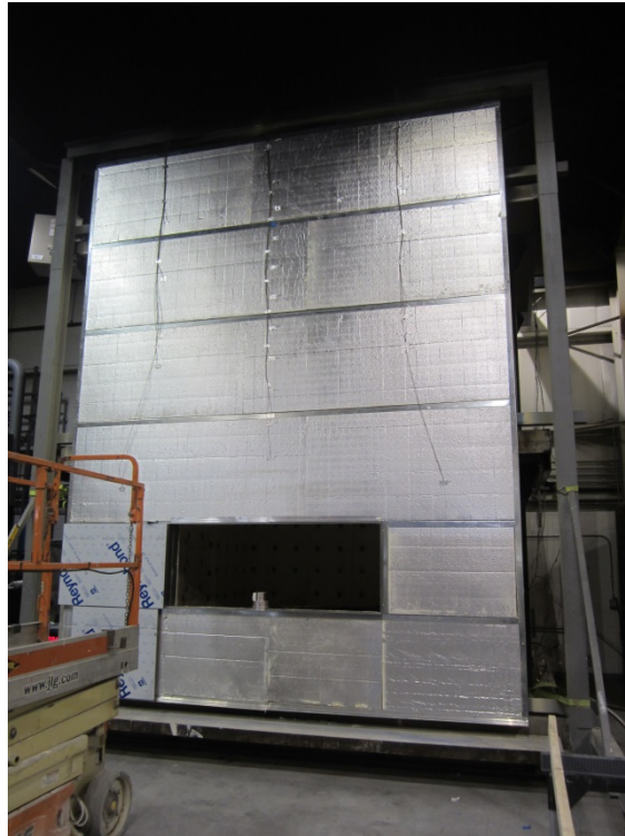
Photo No. 7 Complete Insulation Installation
