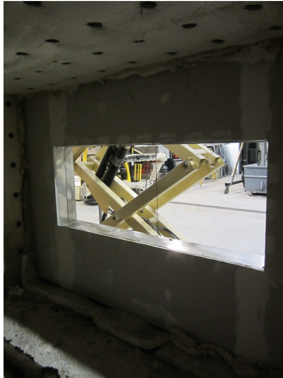
Photo No. 11 First Story Interior (Pre-Test)
