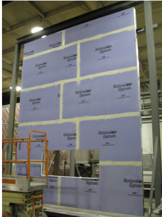
Photo No. 1 Sheathing and Application of Joint System
