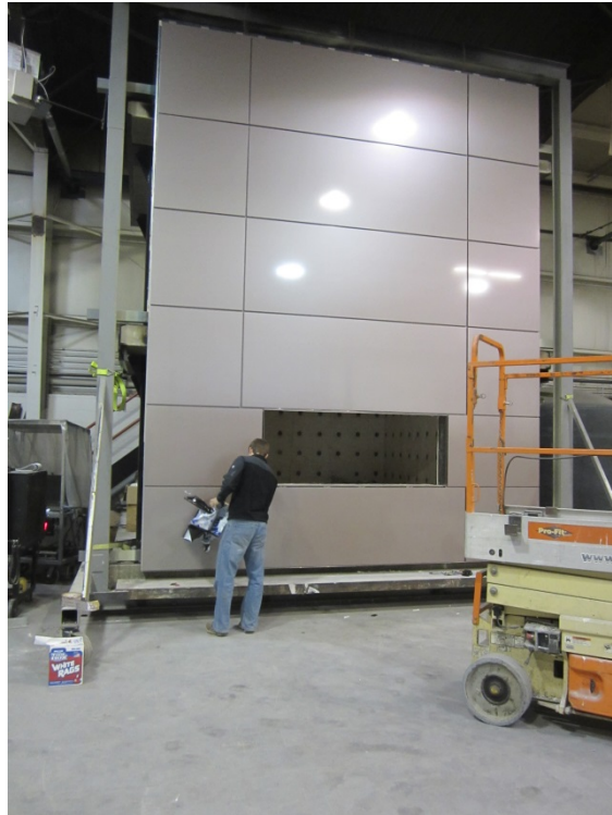
Photo No. 9 Panel Installation Complete
