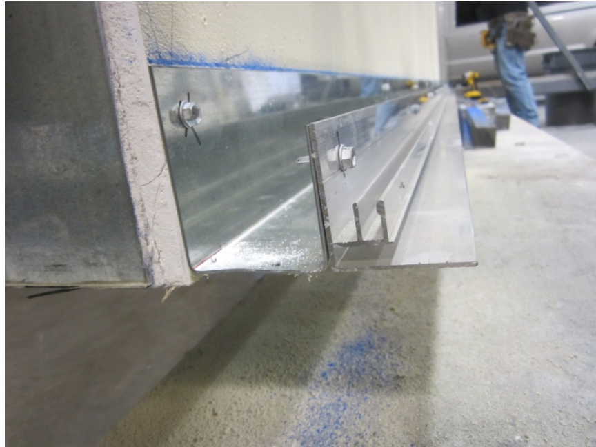
Photo No. 3 Assembly Sill Flashing and Starter Rail
